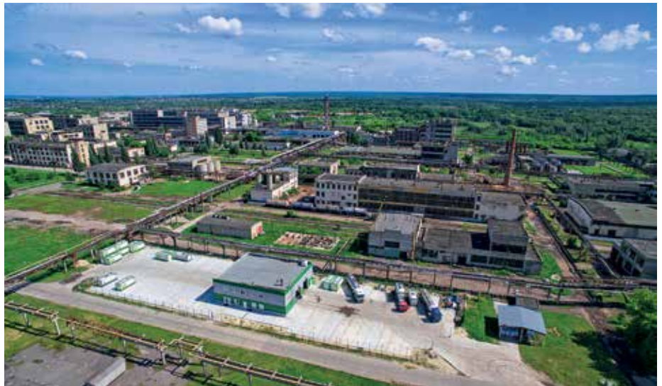
Havila's tank cleaning operation in Tambov, some 450km southeast from Moscow
